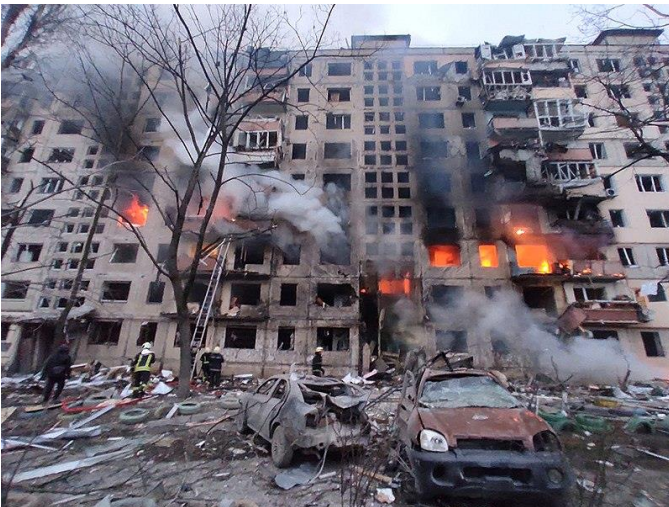
House on Bohatyrskya Street, Kyiv after shelling of 14 March 2022, https://cs.m.wikipedia.org/wiki/Soubor:House_on_Bohatyrskya_Street_after_shelling_of_14_March_2022_(01).jpg
